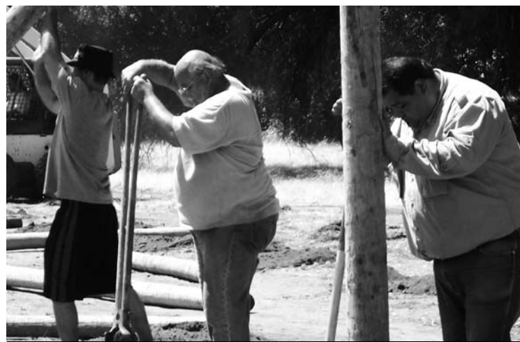
Barona Tribal member Steve Banegas (right) with Vice Chairman Beaver Curo and Museum intern Paul Jeffrey planting the posts that will support the ramadas at the Gathering grounds. Photo by Cheryl Hinton.
